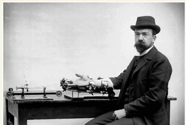
Figure 7 Angelo Mosso performing one of his experiments. Here Mosso is photographed with his pneumograph at pneumatic transduction with two drums, an evolution of Marey's pneumograph, which in contrast had only one drum with a flexible guttapercha membrane (courtesy of Marco R. Galloni).
